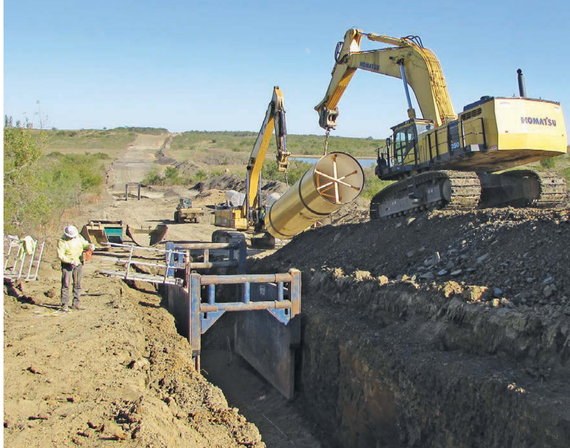
Clockwise: A crew from the Tarrant Regional Water District works inside a shoring box on a section of the 150-mile-long water supply pipeline currently under construction; crews use large excavators to lower a section of the new water supply pipeline into the trench; crews move a section of the new line into place for connection.
