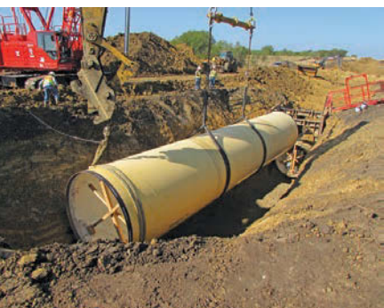
Clockwise: A crew from the Tarrant Regional Water District works inside a shoring box on a section of the 150-mile-long water supply pipeline currently under construction; crews use large excavators to lower a section of the new water supply pipeline into the trench; crews move a section of the new line into place for connection.
