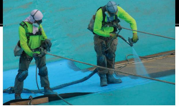
The contractor's crew sprayed polyurea on all stairs, sumps and penetrations at the reservoir, and then tied those to the geotextile.
