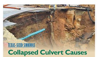
Heavy rainfall led to the washout of a stormwater culvert in Granburgy, Texas, creating a massive sinkhole — and a \$500,000 problem — for the City. After surveying the damage left by the 45-footwide, 30-foot-deep crater, it was discovered that sewer lines attached to a nearby pumping station were severed and the lift station itself was a total loss. Learn how city crews helped minimize the discharge of wastewater into local waterways, allowing for repair efforts to begin. mswmag.com/ featured
