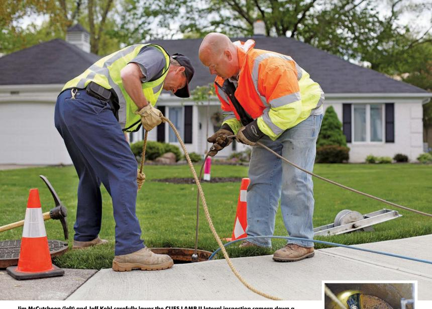
Jim McCutcheon (left) and Jeff Kohl carefully lower the CUES LAMP II lateral inspection camera down a manhole. Right: The camera is positioned at the bottom of the manhole for entry into the pipe.
