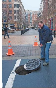
Rockville Department of Public Works crew members Larry Connelly (left) and Randy Maness set up to flush a sewer main. Right: Engineer technician Joel Karpas removes a manhole prior to an acoustic line inspection.
