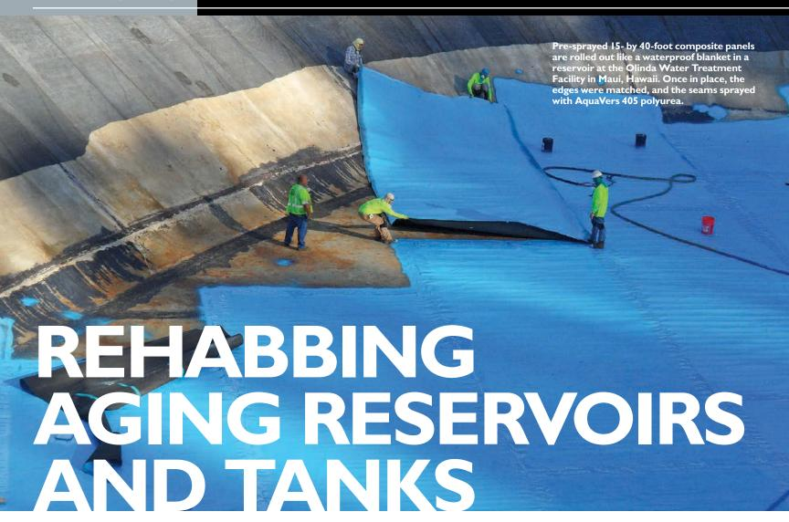
Advanced polyurea coatings and liners provide strong, flexible waterproofing capable of bridging large cracks
