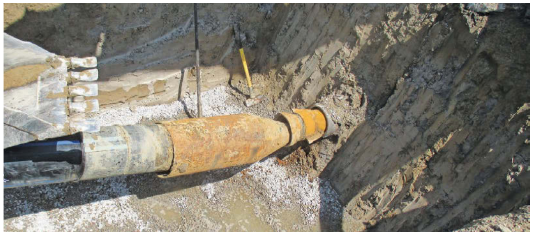
The tool string consists of the pull rod (inside the pipe at this point) connected by a flex joint connector to the pulling head. The pulling head is nestled inside the expander, which drives the splitter (seen here positioned at the pipe mouth).
