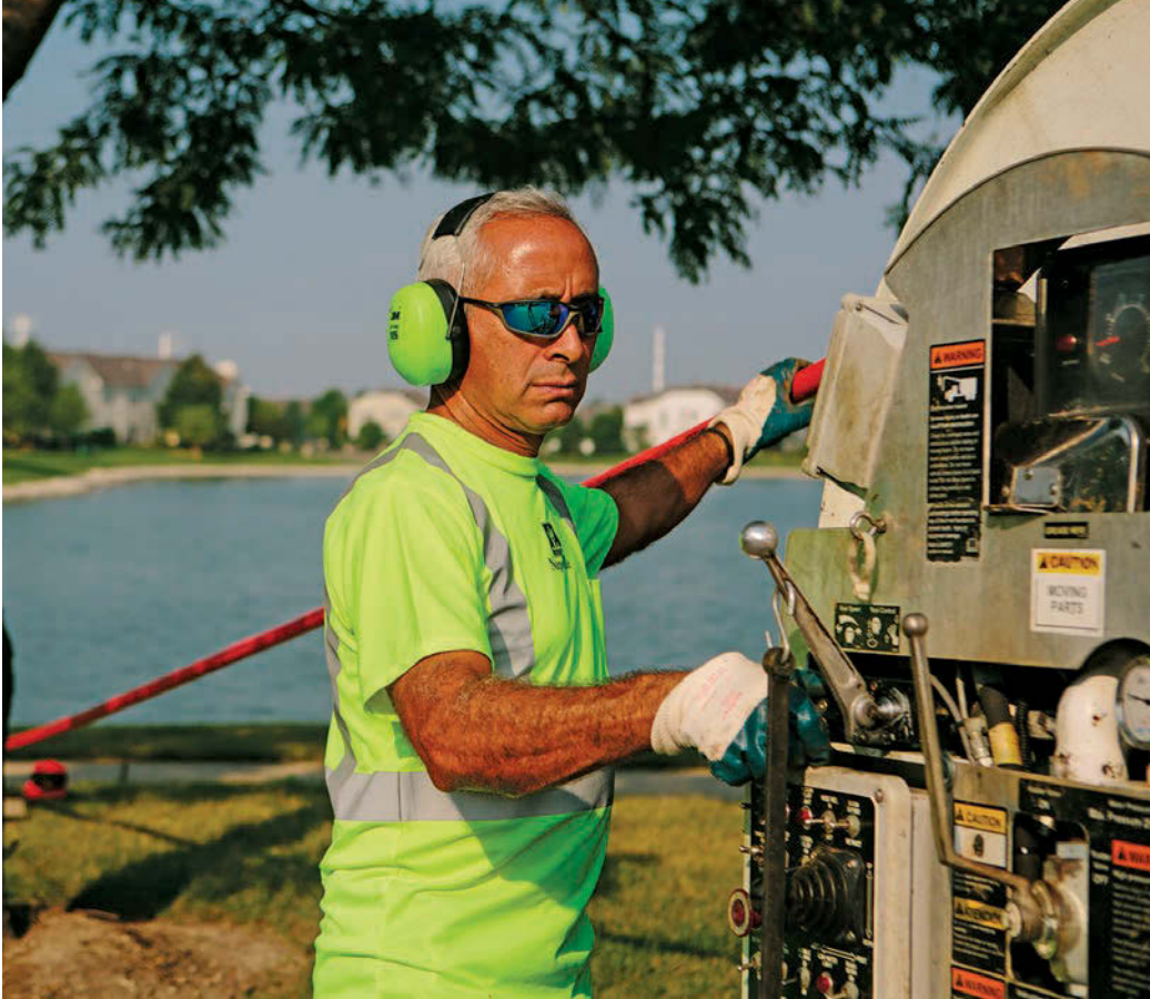
Left: Dino Tinajero operates the controls on a Vactor combination truck while cleaning a sanitary sewer line in a newer residential development. Above: Utility technician Steve Subat operates the truck's jetting system remotely while flushing a sewer main.
