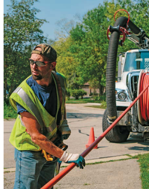
Left: Dino Tinajero operates the controls on a Vactor combination truck while cleaning a sanitary sewer line in a newer residential development. Above: Utility technician Steve Subat operates the truck's jetting system remotely while flushing a sewer main.
