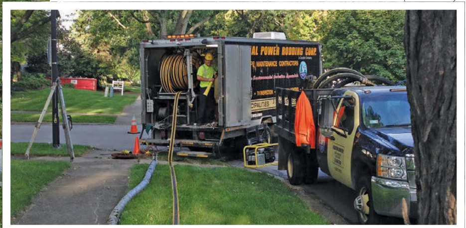
A National Power Rodding crew member lubricates a Logiball lateral packer at the start of a grouting job in Naperville, Illinois. Right: The five-line grouting hose includes two air lines, one vacuum line and one line for each of the two grout components.
