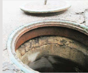
Concrete ADJ Rings Installed 1997
