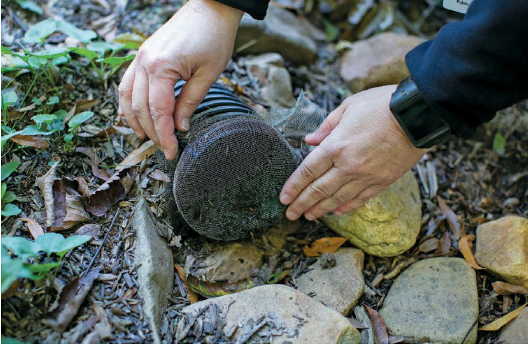
Civil engineer Sandi Wilbur checks an output tube in one of 40 rain gardens that were installed to catch rainwater runoff and prevent flooding. The tube runs from the base of the house where rainwater is caught to the rain garden at the bottom of the hill. Right: A water level indicator shows that the creek bed is only 7 inches deep near the South Ellerbe Creek water monitoring station. The Rain Catchers program is aimed at trapping some of the water in yards instead of flowing straight to the creek.
