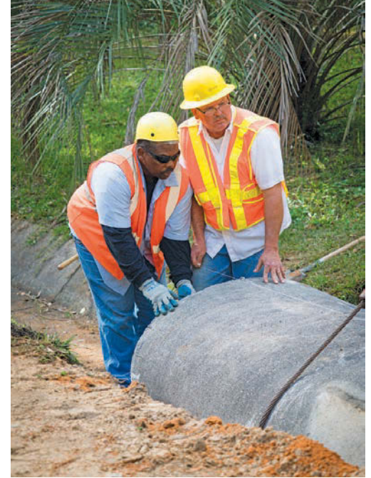
ABOVE: Erasmo Mendoza and Facundo Mendoza of Allen's Excavation work on a City of Tallahassee water replacement project. RIGHT: Terry Plummer (left) and Paul Davis help align a new piece of concrete pipe that is replacing the old open-ditch stormwater system.
