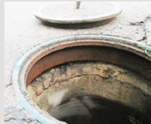
Concrete ADJ Rings Installed 1997
