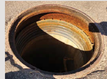
Ladtech ADJ Rings Installed 1997
