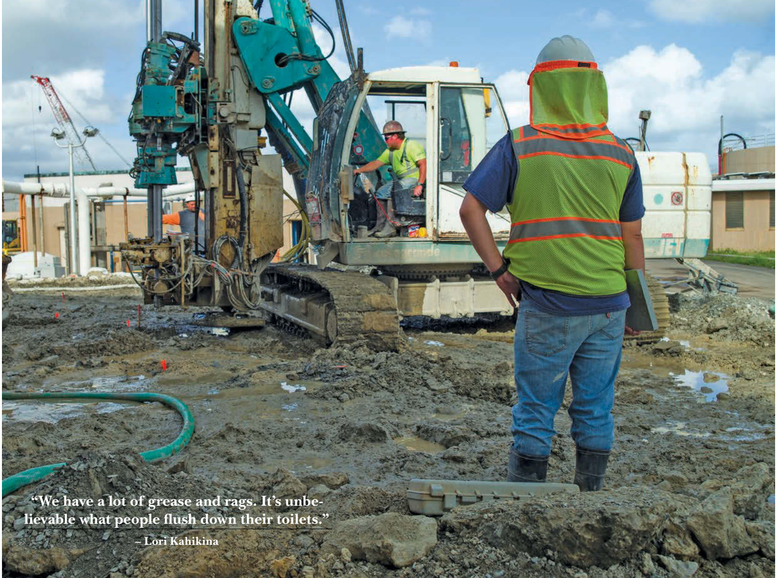
Above: Workers pump grout around the Mokapu diversion structure at the Kaneohe-Kailua Tunnel project in Kaneohe. Left: A crew member inspects the area around the secondary odor control fan housing and ducts outside the tunnel.
