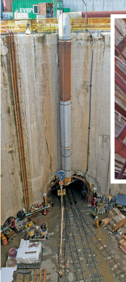
Left: Workers stage materials and equipment in the entrance shaft outside the Kaneohe-Kailua Tunnel project in Kaneohe, Hawaii. Above: A construction crew works on the drop structure where excess flow from Kailua is directed into the tunnel.
