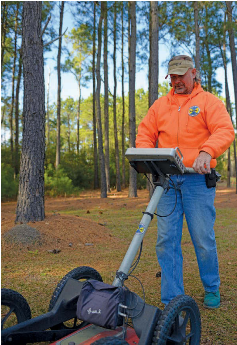
Robert Horn uses the MALA GPR unit to locate underground utilities in a wooded area along the edge of a subdivision.
