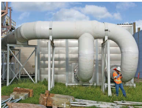
Above: Workers pump grout around the Mokapu diversion structure at the Kaneohe-Kailua Tunnel project in Kaneohe. Left: A crew member inspects the area around the secondary odor control fan housing and ducts outside the tunnel.
