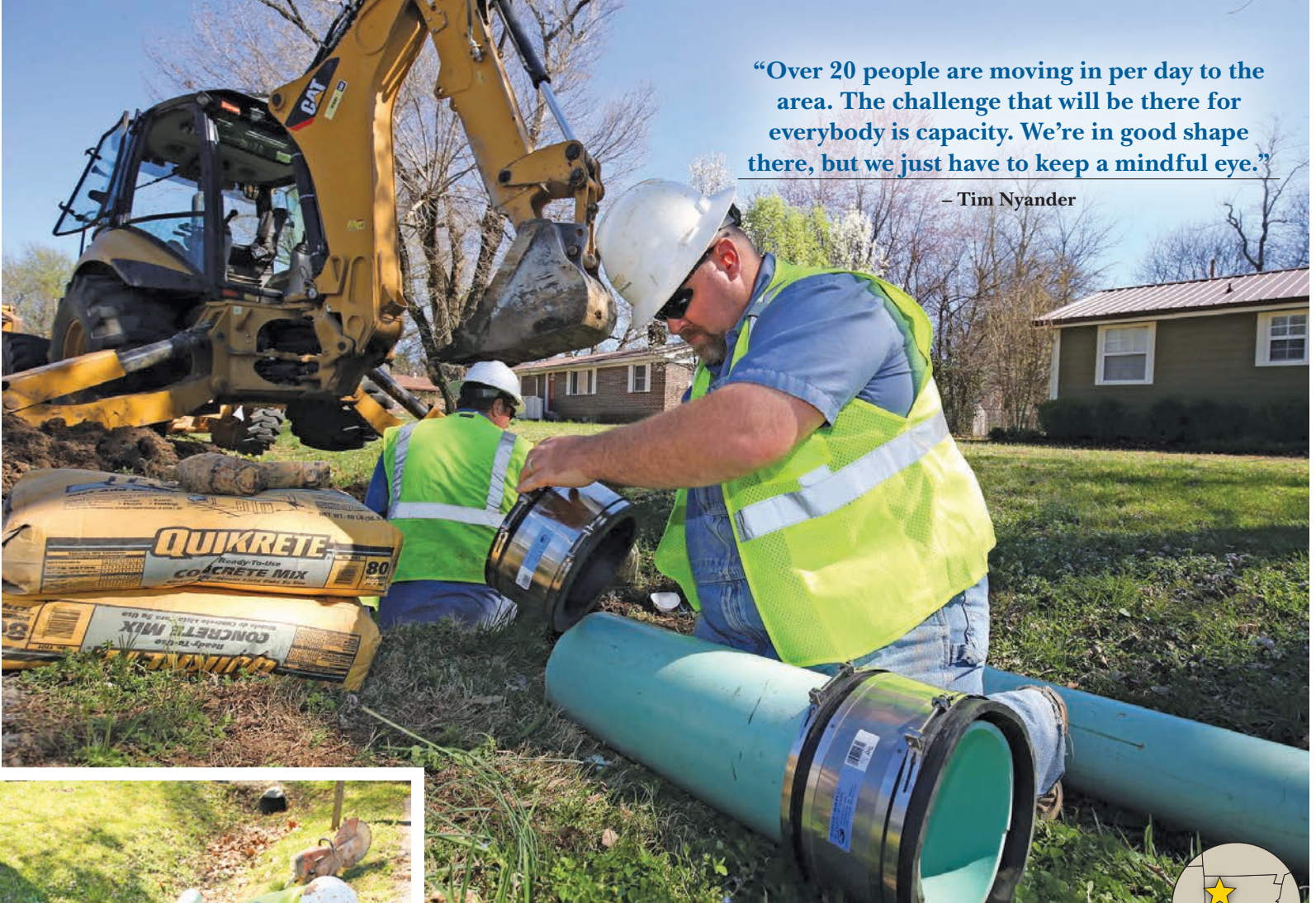
Above: Wayne Smith of Fayetteville Water & Sewer Utility attaches Fernco couplings to a piece of 8-inch pipe for a sewer line repair. Left: Charlie Thompson, Matthew Childers and Smith (from left) install the replacement pipe.
