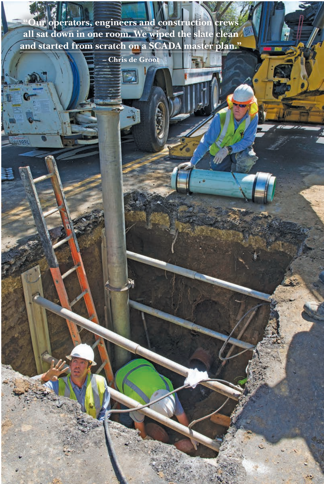
Left: Maintenance workers repair a damaged section of sewer main in the middle of a residential street while a Vac-Con jet/vac truck keeps the pit dry. Above: Justin Pinheiro cuts a new piece of pipe for a sewer main repair.
