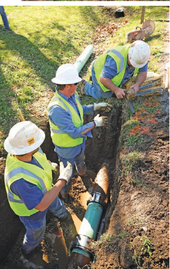
Above: Wayne Smith of Fayetteville Water & Sewer Utility attaches Fernco couplings to a piece of 8-inch pipe for a sewer line repair. Left: Charlie Thompson, Matthew Childers and Smith (from left) install the replacement pipe.
