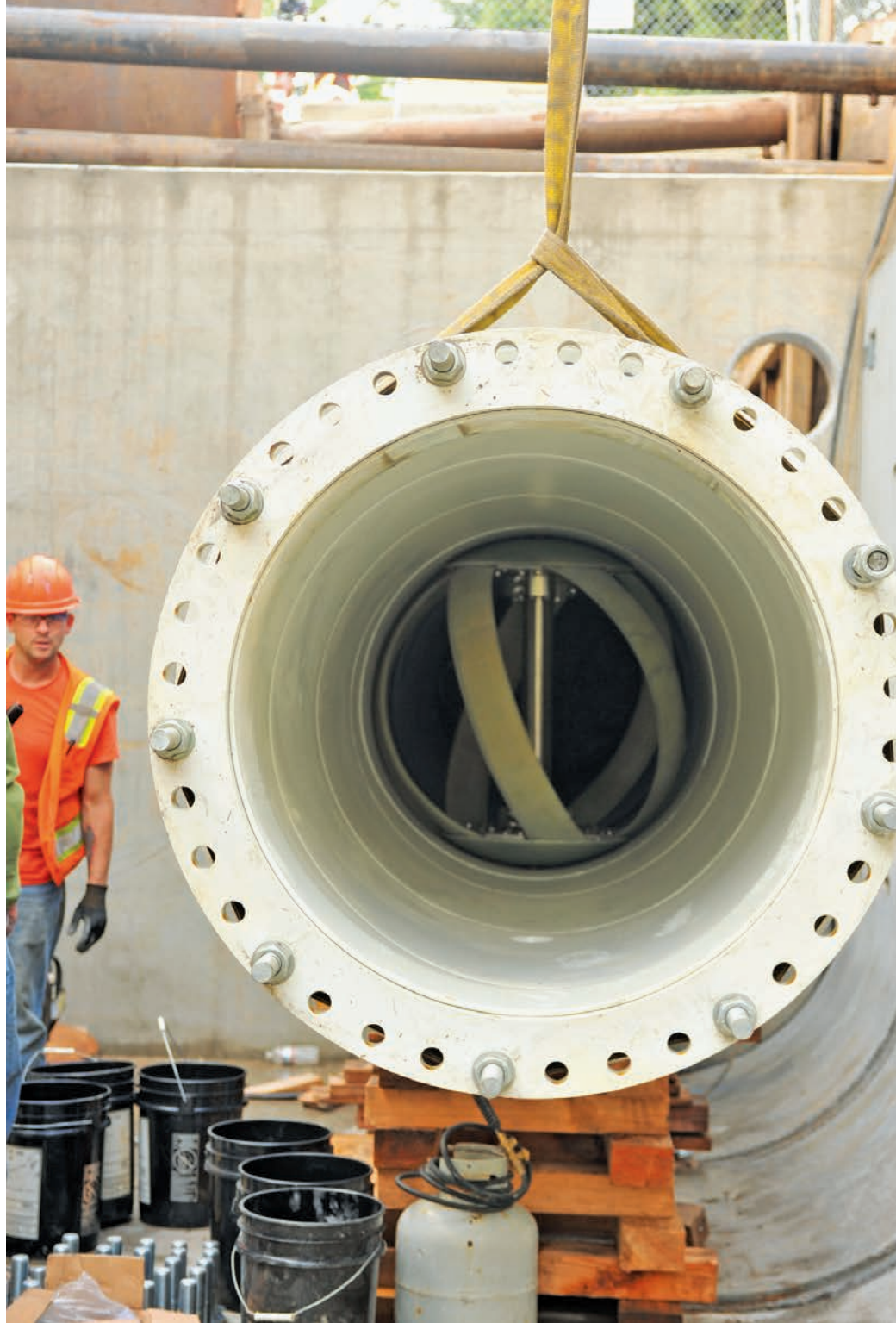
LEFT: Four turbines were installed across 50 feet of a 42-inch gravity-fed pipe, producing enough electricity to power up to 150 homes for a year. (Photo Sherri Kaven) ABOVE: The LucidPipe turbine requires flows of at least 20 cfs at 40 psi. Each turbine also acts as a pressure reduction valve, reducing head pressure by 1 to 5 psi. (Photo Lucid Energy)
