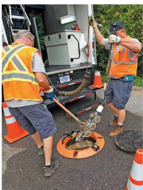
Mike Jones (left) and Gary Cantrell lower a CUES camera through a Light Ring into a manhole for a sewer line inspection.
