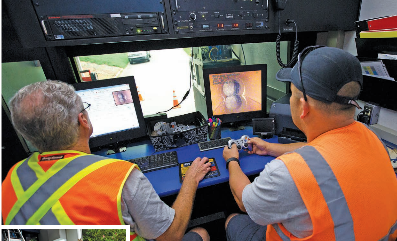
Technician Mike Jones (left) and TV crew leader Gary Cantrell run a sewer line inspection from the control room of the CCTV van.
