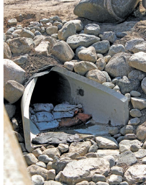
This 36-inch stormwater outfall along the Wisconsin River on the edge of downtown Rhinelanders is the smaller of two new outfalls that replace a lone 24-inch outfall.
