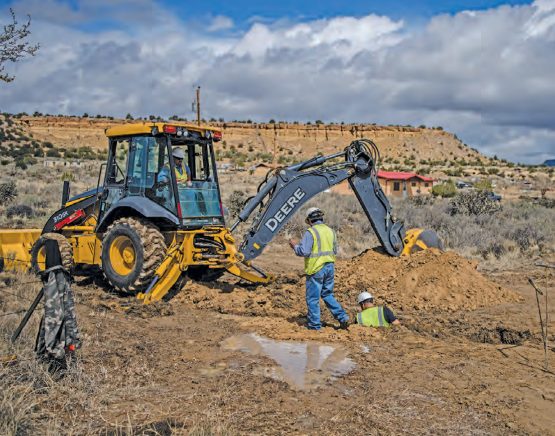
Left: Water and wastewater department employees excavate a water main to add new connections for nearby homes. Right: Limbert Martinez uses a Wacker Neuson soil compactor near a newly installed septic tank at a new office in the Pueblo of Acoma.
