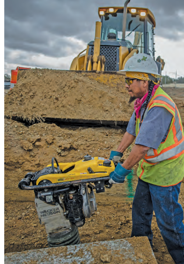
Left: Water and wastewater department employees excavate a water main to add new connections for nearby homes. Right: Limbert Martinez uses a Wacker Neuson soil compactor near a newly installed septic tank at a new office in the Pueblo of Acoma.
