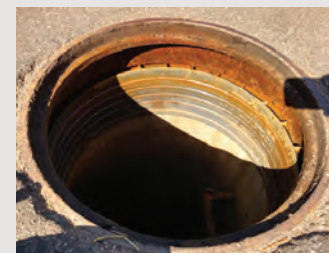
Ladtech ADJ Rings Installed 1997
