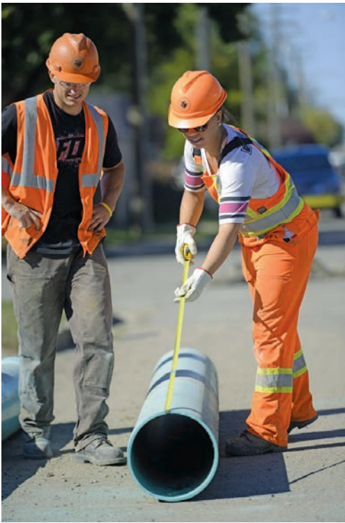
Pipefitter Mel Patoine measures a length of storm sewer pipe with Clayton Hall.
