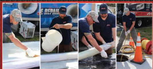
SECTIONAL POINT REPAIR
