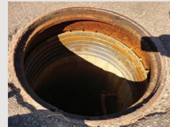
Ladtech ADJ Rings Installed 1997
