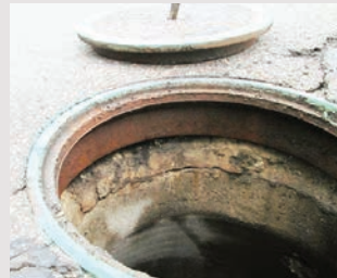
Concrete ADJ Rings Installed 1997
