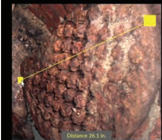
Measureable Point Cloud
