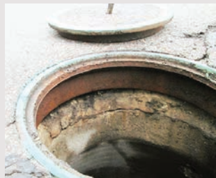
Concrete ADJ Rings Installed 1997
