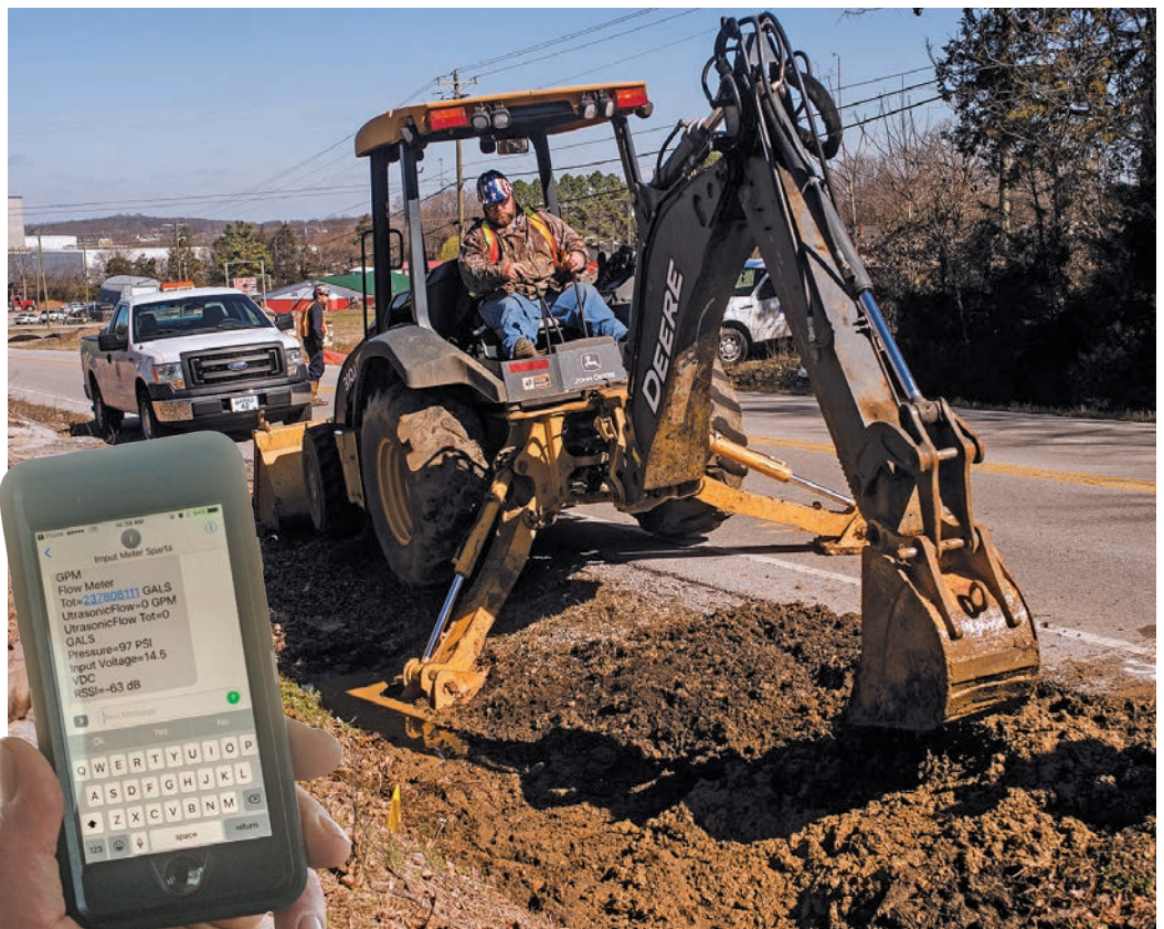
Left: B.J. Baugus does a remote check on a flow meter from his smartphone. Above: Andy Adsmond uses a backhoe to backfill around a pipe after repairing a leak.
