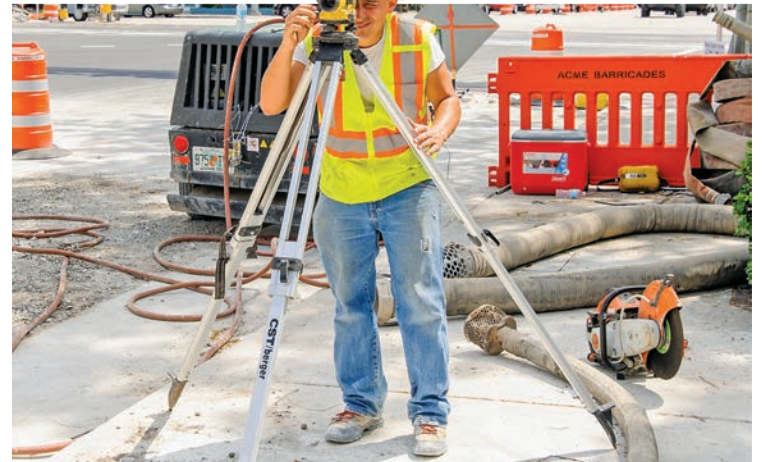
Clockwise from top: Crew members prep a section of pipe for installation. The new 48-inch force main is part of the N. Miami Avenue Betterment Project; Contractor foreman Cody Cook uses a TopCon level to shoot grades for the new pipe; A hydraulic pump is loaded onto a flatbed truck along N. Miami Avenue.
