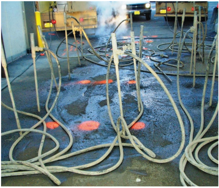
Above: A steam set thaws the ground so work on a water main can begin.
