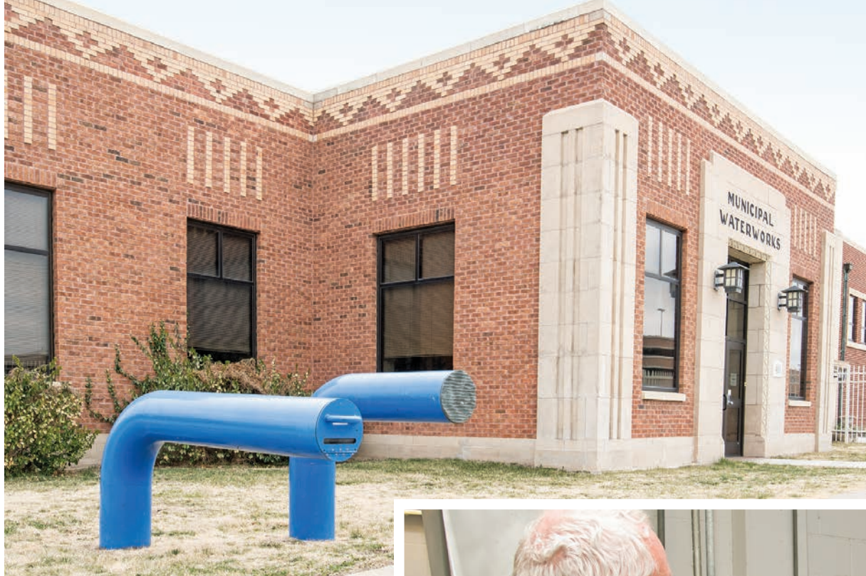
Left: A general view of the exterior of the Municipal Waterworks plant in Salina, Kansas. Below: Plant employee Mark Peterson and Director Martha Tasker examine the chemical feed system provided by Merrick.
