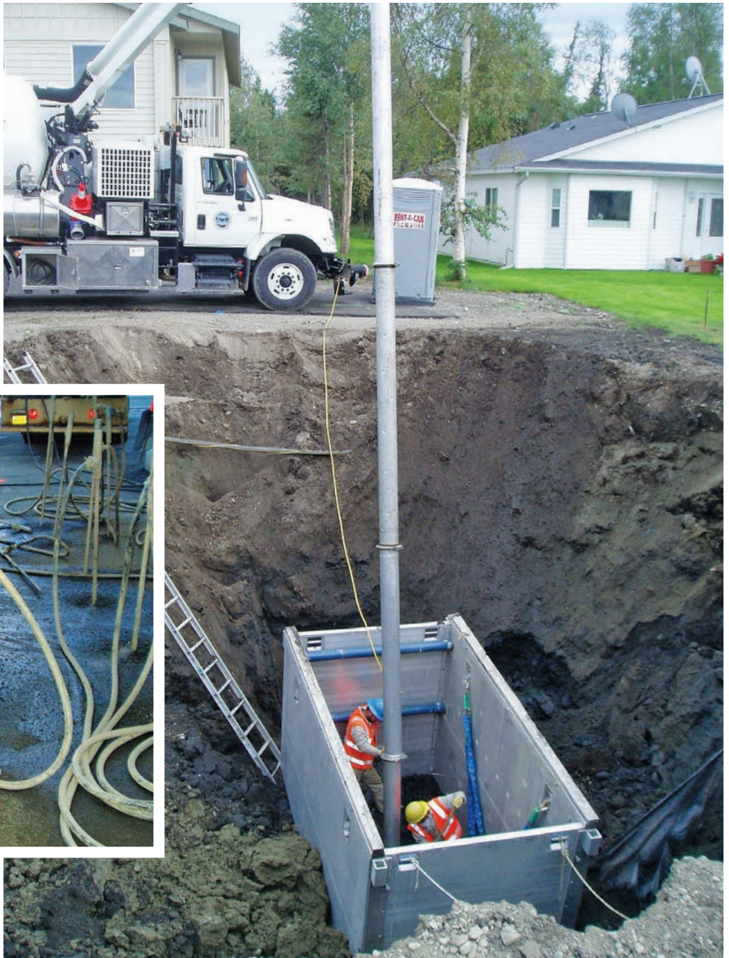
Above: A steam set thaws the ground so work on a water main can begin.
