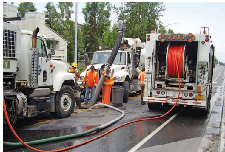
Crew members clean a line.
