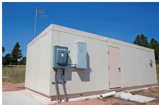
The Southern Black Hills Water System's Junction Booster Station is one of three such stations that help maintain pressure across a 1,500-foot system elevation variance.
