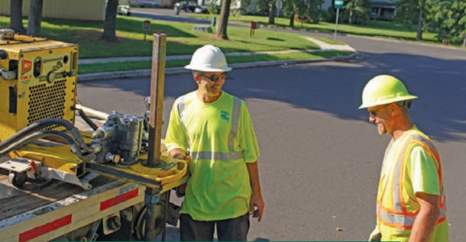
John Myers (left) and Rob Averitt exercise water system valves in a residential neighborhood using a Wachs TM-7 valve exerciser.
