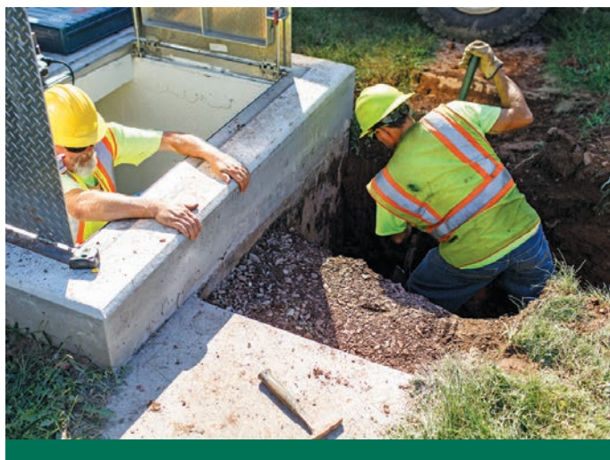
Erwin Hunsberger (left) and Angelo Cosentino work on a 3/4-inch sample service for the Lawn Avenue storage tank.
