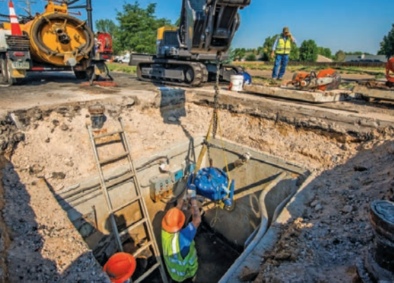
Members of the Greeley water crew lower and place a new pressure release valve in an existing vault.
