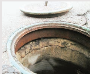
Concrete ADJ Rings Installed 1997
