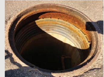
Ladtech ADJ Rings Installed 1997
