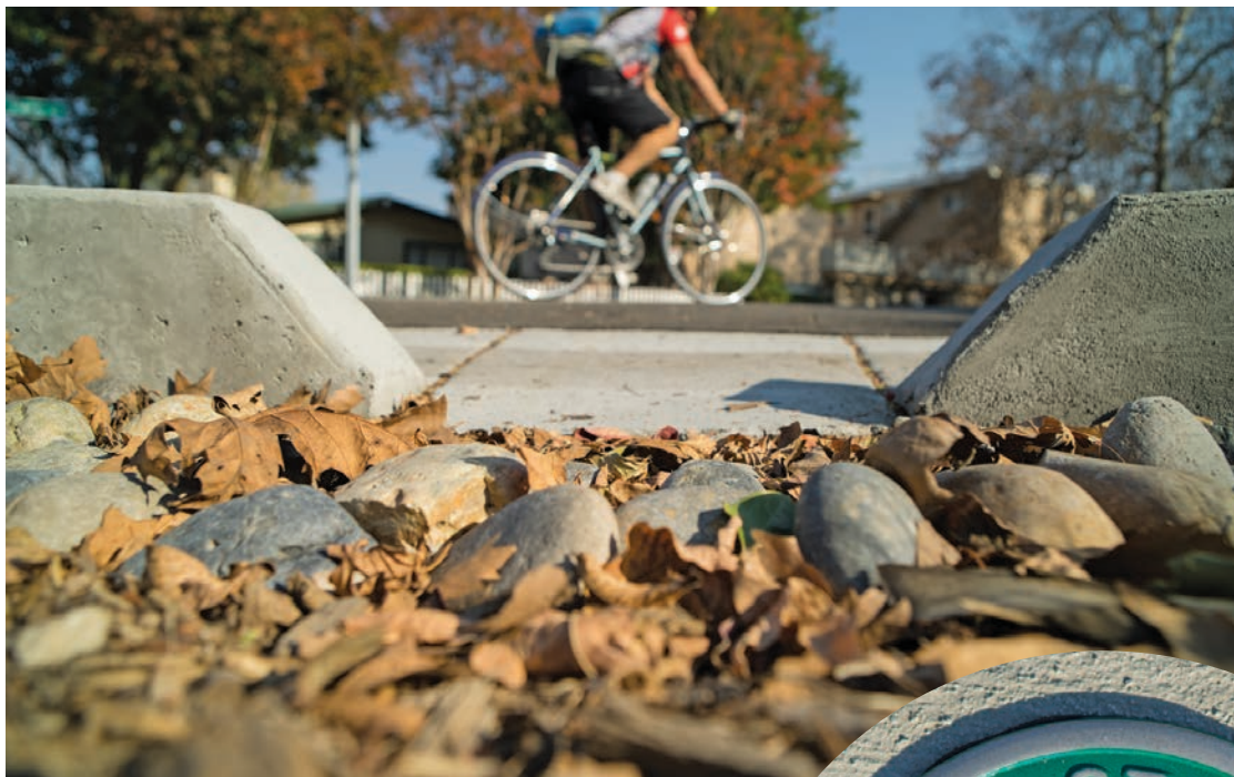
A cyclist speeds past a stormwater collection point on Park Avenue in San Jose. The green stormwater features have beautified local roadways and improved safety by eliminating pooling runoff water.
