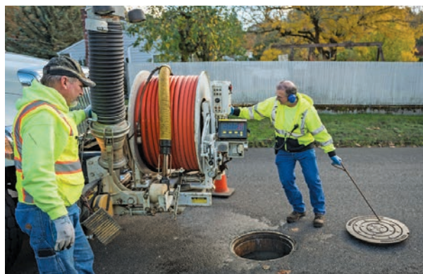
Dean Ronk replaces a manhole cover after using a Camel jet/vac truck to clean the sewer line.
