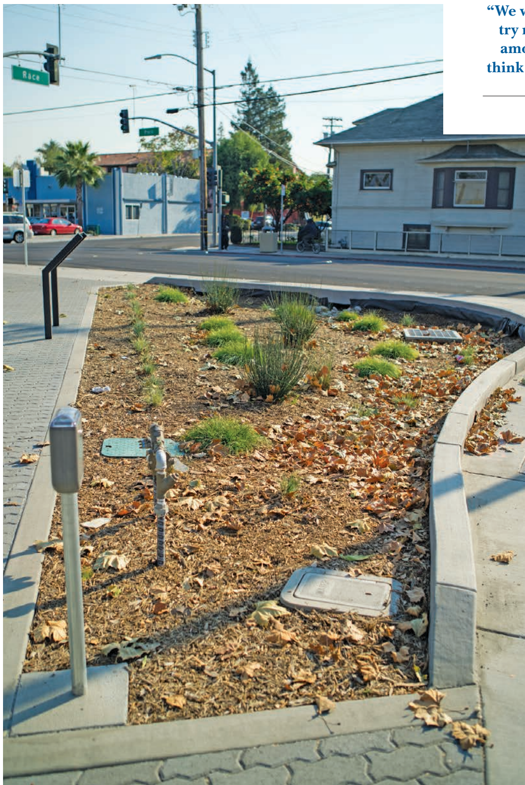
In November, San Jose completed work at four intersections on Park Avenue. Asphalt was replaced with permeable pavement and curbside rain gardens.
