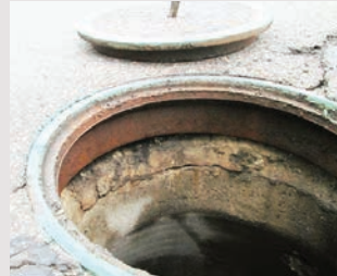
Concrete ADJ Rings Installed 1997
