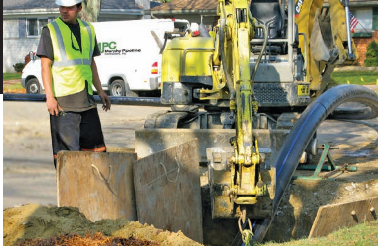
A crew member works at the entry pit, guiding new HDPE into the host pipe on a prechlorinated pipe bursting job.
