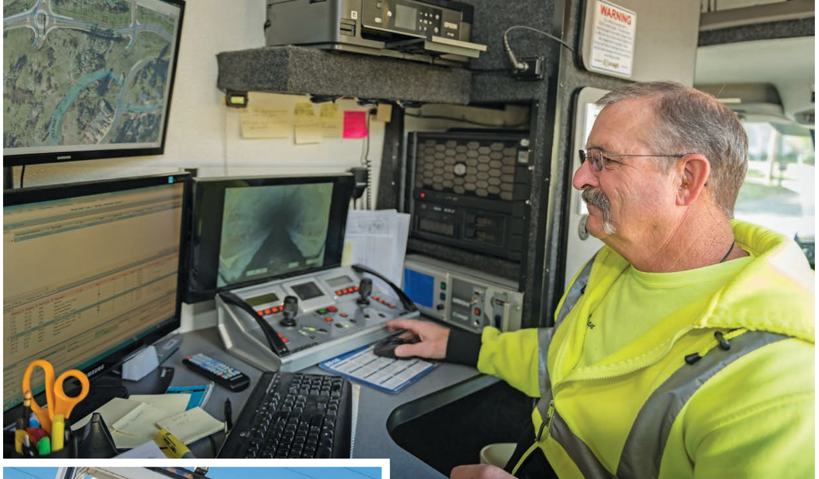
Above: Dean Ronk sits at his operator's station, monitoring the camera's progress and coding defects during a sewer line inspection. Left: Ronk washes of an EnviroSight camera and transporter after completing the inspection.
