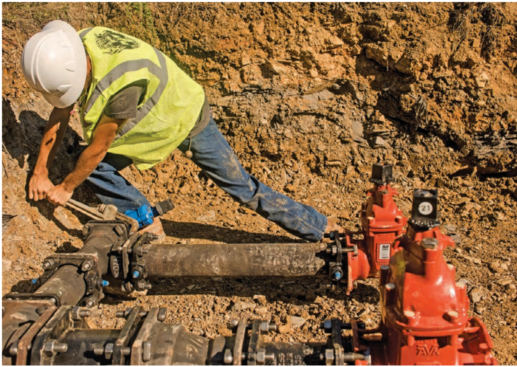
A Kingsport Water Service worker connects a valve on a new AVK water meter.
