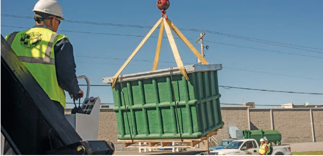
A water meter vault is lifted from a boom truck to be set in place at a new construction site.
