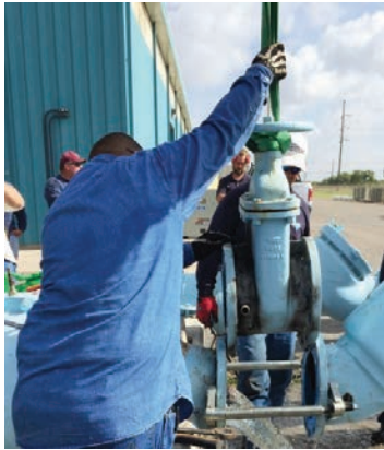
Spread outside flanges & remove old valve
