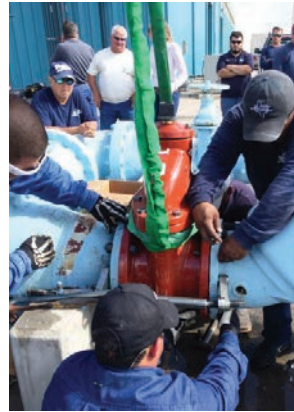
Reinstall new valve
