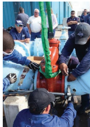
Reinstall new valve
