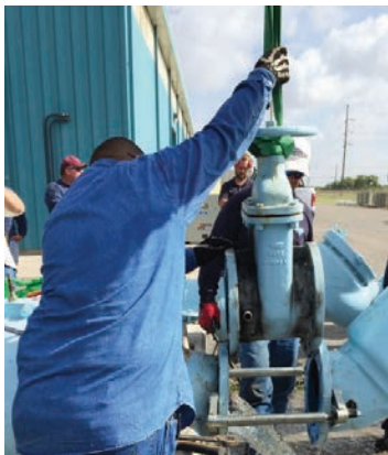
Spread outside flanges & remove old valve
