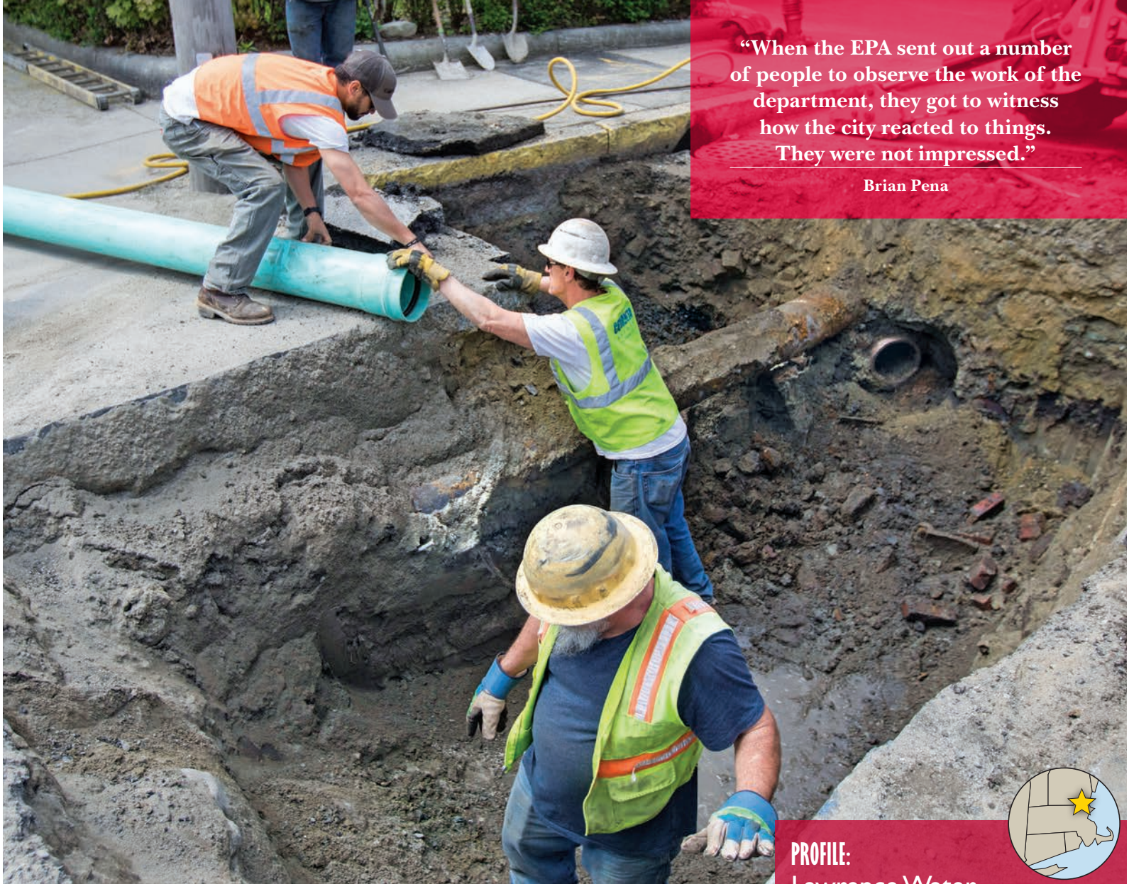
Sewer & Water Department workers Eddie Santiago (left) and Frank Rapisardi move a length of polyvinyl chloride pipe into place to replace a crushed drainage pipe while Frank Condo readies himself in the pit.
