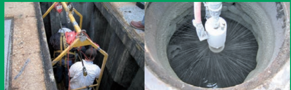
REHAB WITH AP/M PERMAFORM & CONSHIELD
