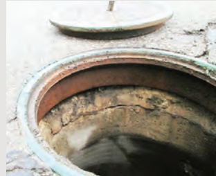
Concrete ADJ Rings Installed 1997
