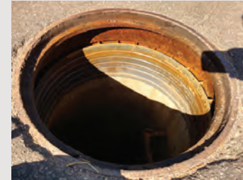
Ladtech ADJ Rings Installed 1997
