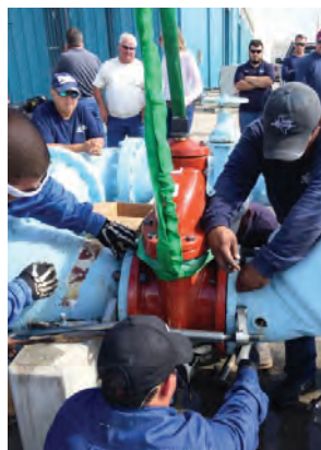
Reinstall new valve
