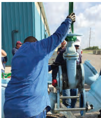
Spread outside flanges & remove old valve
