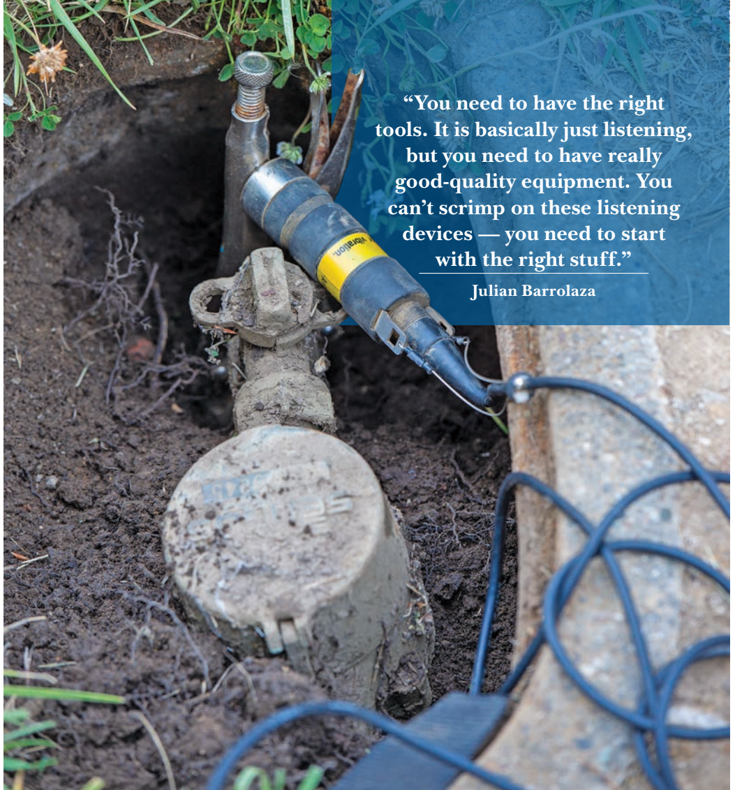
A listening device is connected to waterline as part of the leak detection process.
