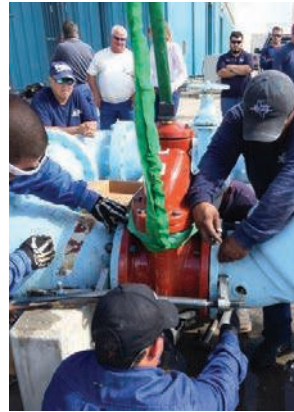
Reinstall new valve
