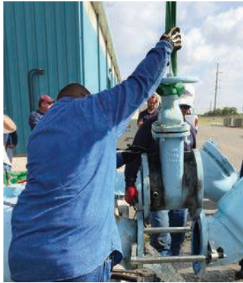
Spread outside flanges & remove old valve
