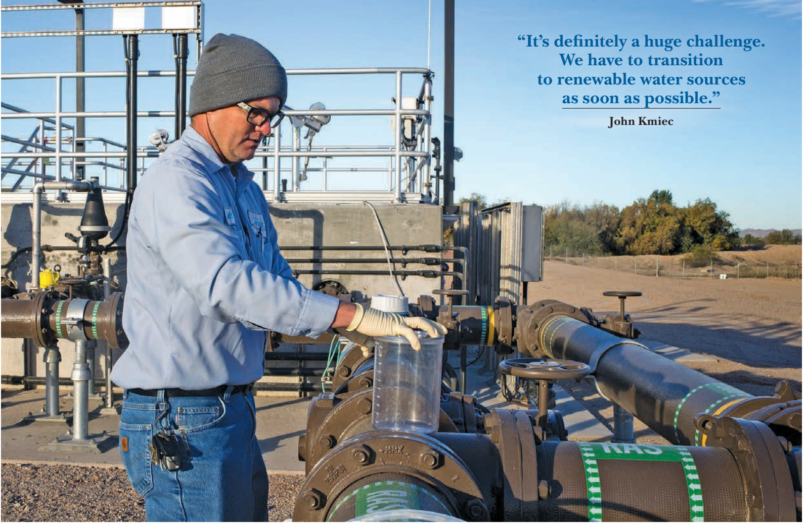
Jeff Smith takes a sample at the Marana Wastewater Reclamation Facility.
