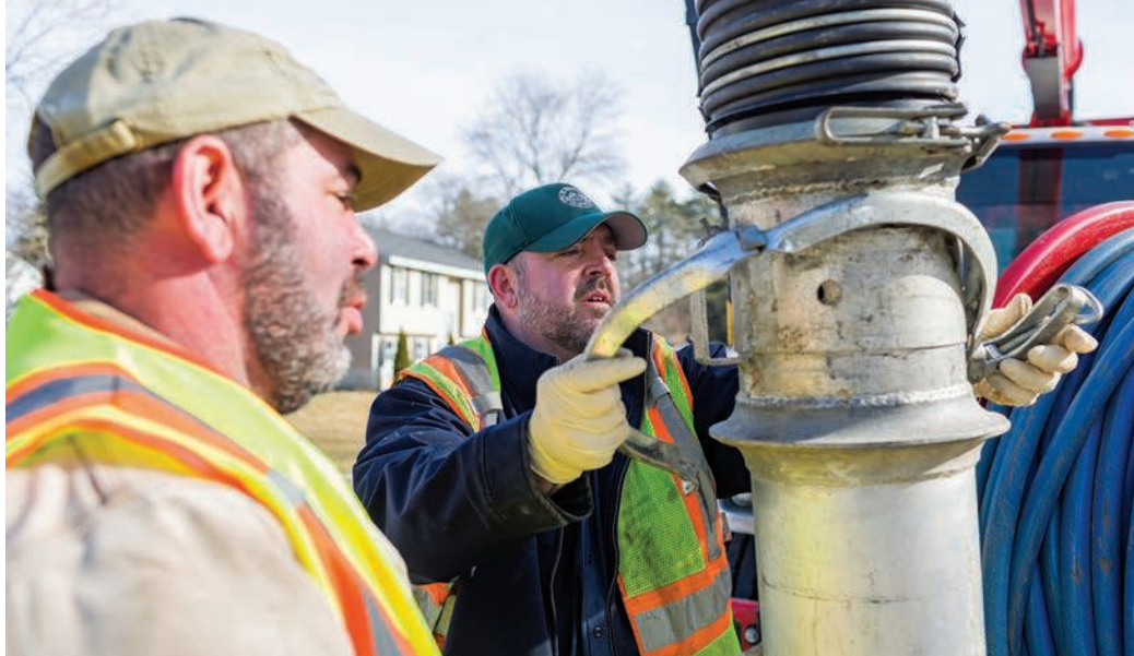
Sam Heffron (left) and Ben Trottier connect the vacuum boom extension to clean debris from a sewer line.
