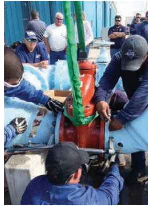
Reinstall new valve
