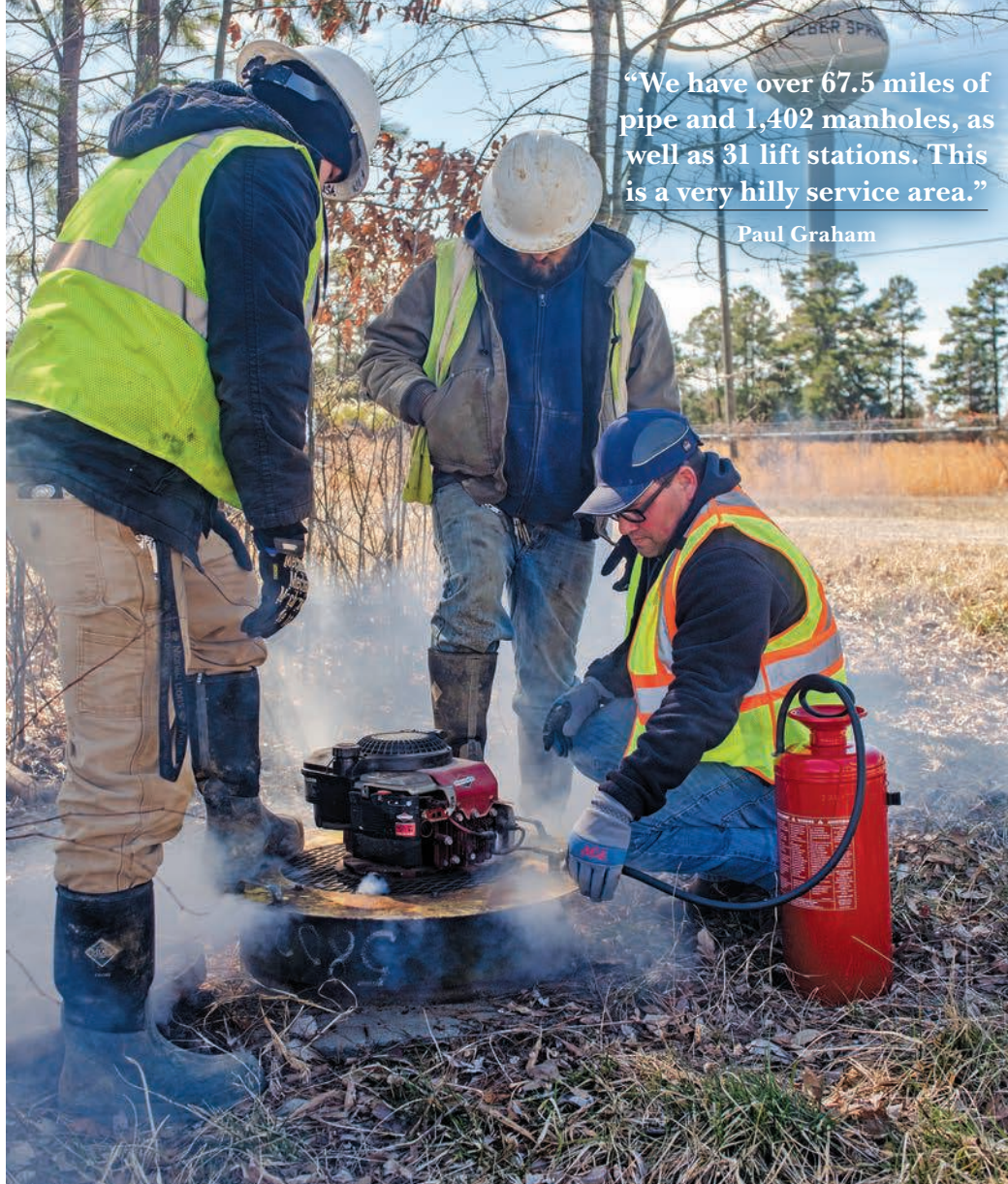
Above: Sewer crew supervisor Brandon Harlan (bottom right) starts a Hurco smoke machine to detect inflow and infiltration in a sewer main. Right: Joey Massey, wastewater treatment plant manager, checks the UV light bulbs on the disinfection system.
