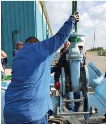
Spread outside flanges & remove old valve
