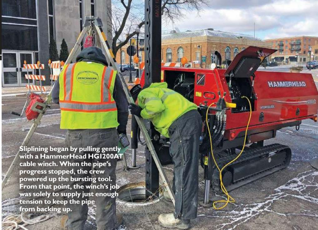
Sliplining began by pulling gently with a HammerHead HG1200AT cable winch. When the pipe's progress stopped, the crew powered up the bursting tool. From that point, the winch's job was solely to supply just enough tension to keep the pipe from backing up.
