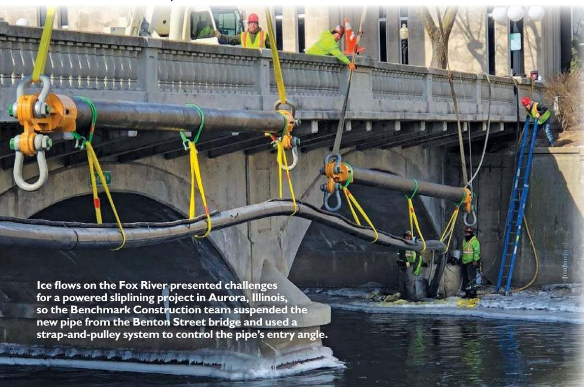
Ice flows on the Fox River presented challenges for a powered sliplining project in Aurora, Illinois, so the Benchmark Construction team suspended the new pipe from the Benton Street bridge and used a strap-and-pulley system to control the pipe’s entry angle.
