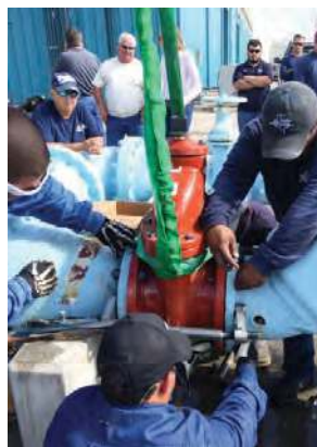
Reinstall new valve
