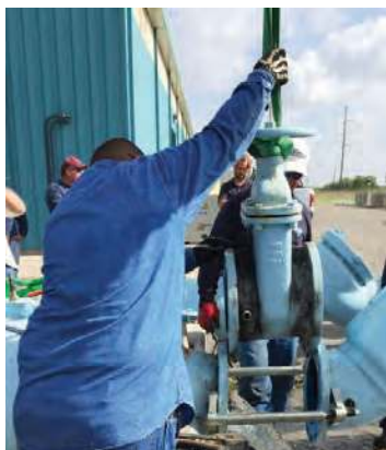
Spread outside flanges & remove old valve
