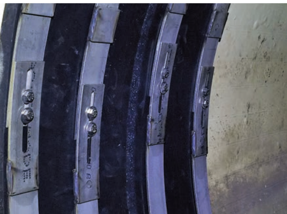
Four stainless steel retaining bands were required on the double-wide seals used on the worst joints.
