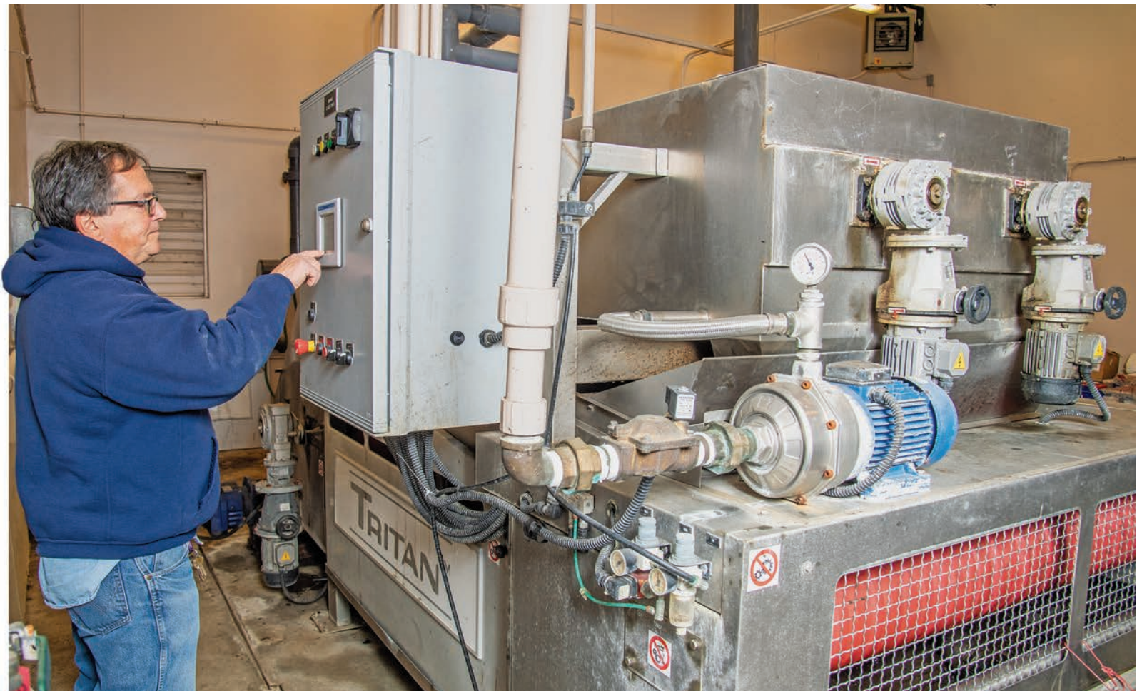
Bonner Springs wastewater collections department supervisor Steve Garcia verifies operation of the Aero-Mod TRITAN belt filter press at the wastewater treatment plant.
