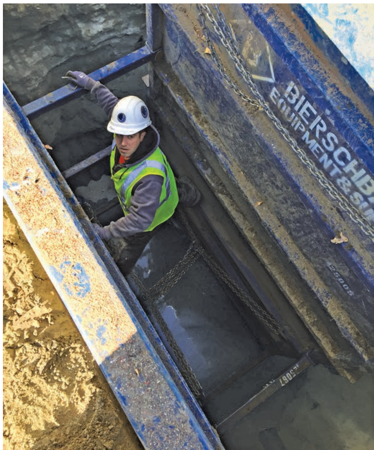
Any trench greater than 5 feet deep must have some type of collapse prevention. The method used for prevention depends on two factors: trench layout and soil conditions.
