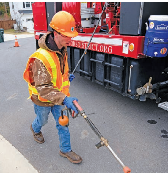
Sewer technician Paul George retrieves an Enz Bulldog Antiblast nozzle to clean a manhole.
