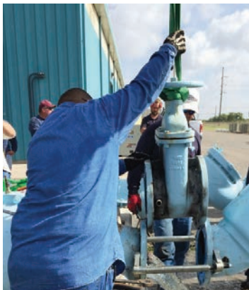
Spread outside flanges & remove old valve
