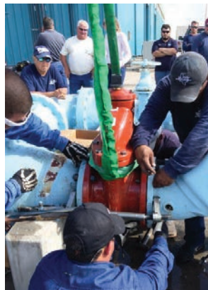
Reinstall new valve
