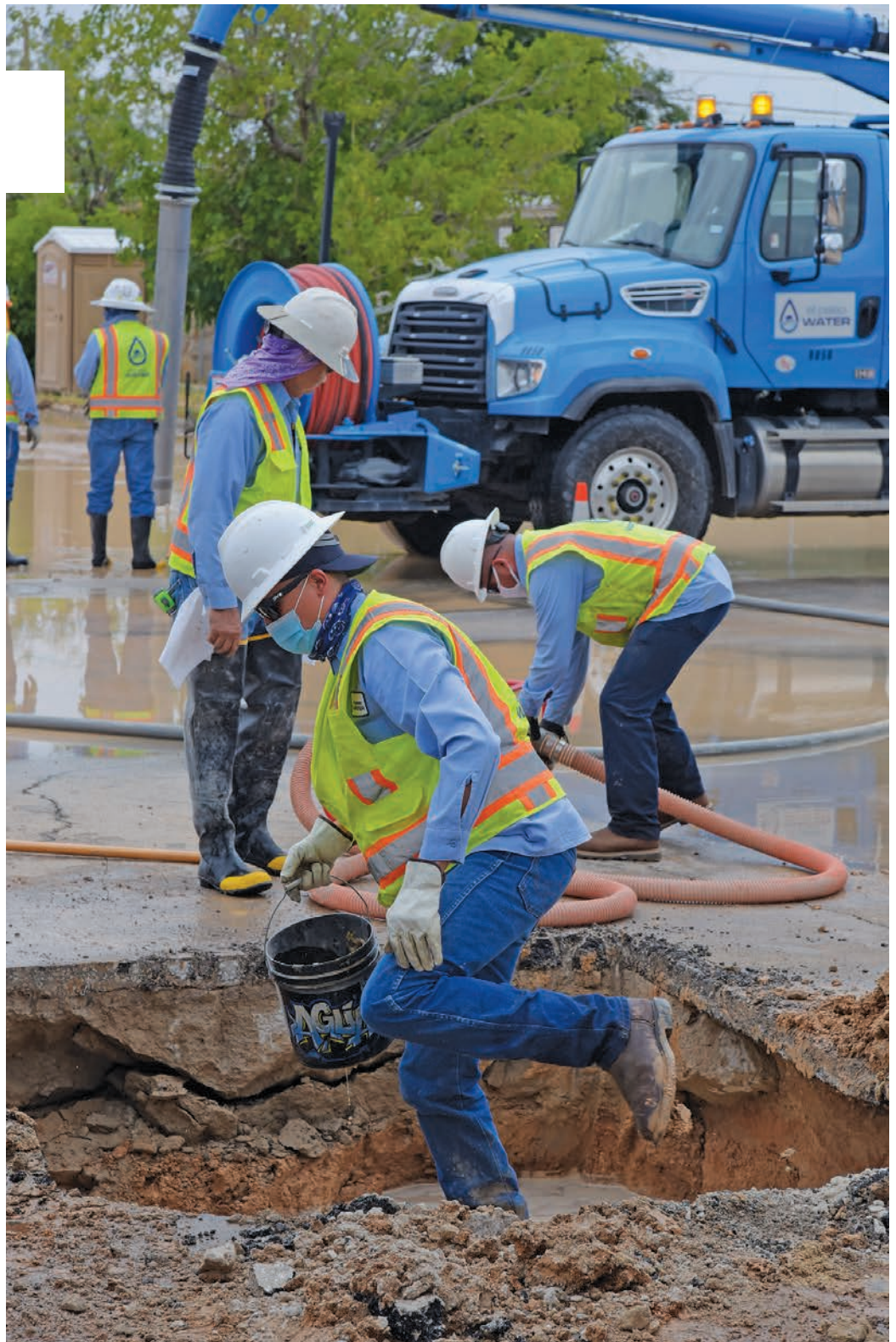
Utility pipe layer Mark Herrera works on the replacement of a broken water main valve.
