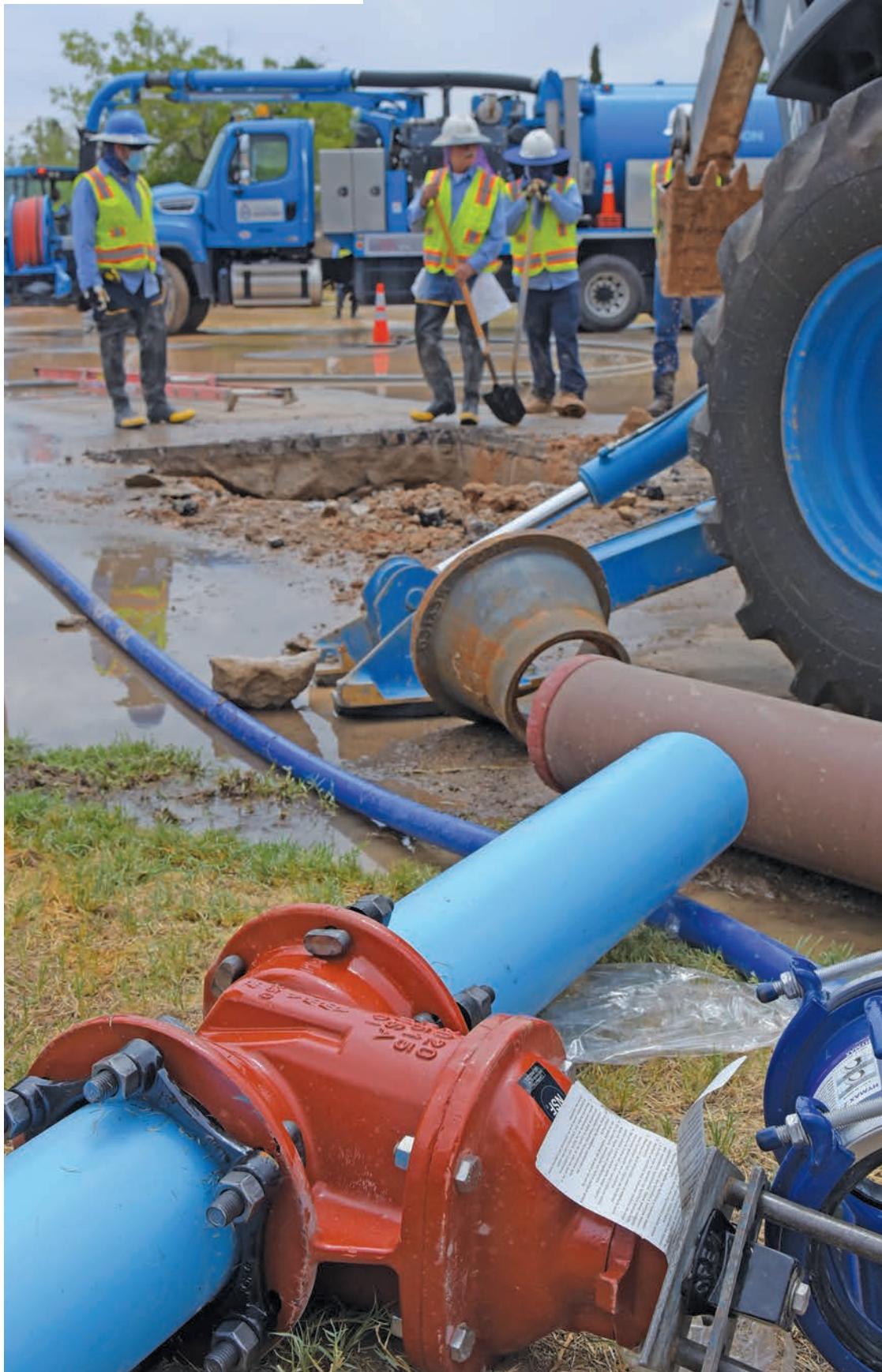
Crew members Marco Munoz, Pascual Rodriguez and Albert Leon (from left) prepare to replace a broken water main valve.
