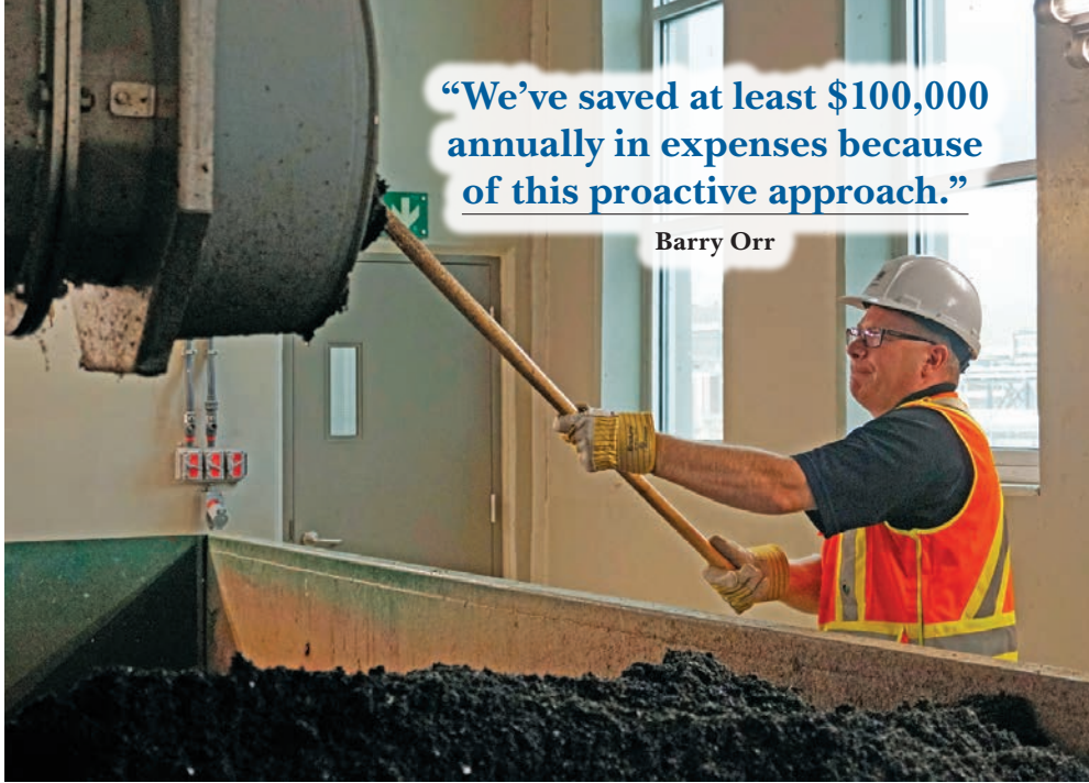
Barry Orr rakes a solids bin at one of the city’s wastewater treatment plants.
