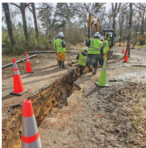
Excavation and replacement of the water line is part of the utility's plan to replace 541 miles of aging, unlined cast iron and galvanized steel pipe.
