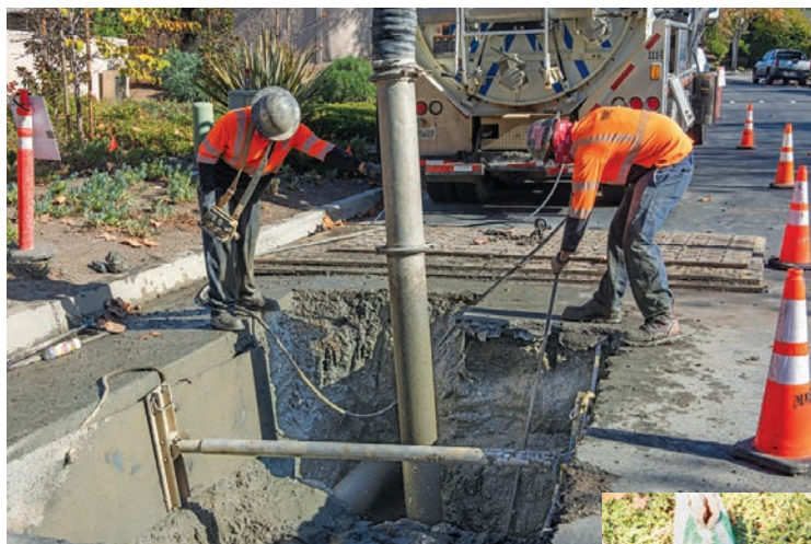
The red valve crew uses a Vactor HXX hydroexcavator to expose a waterline beneath a residential street.
