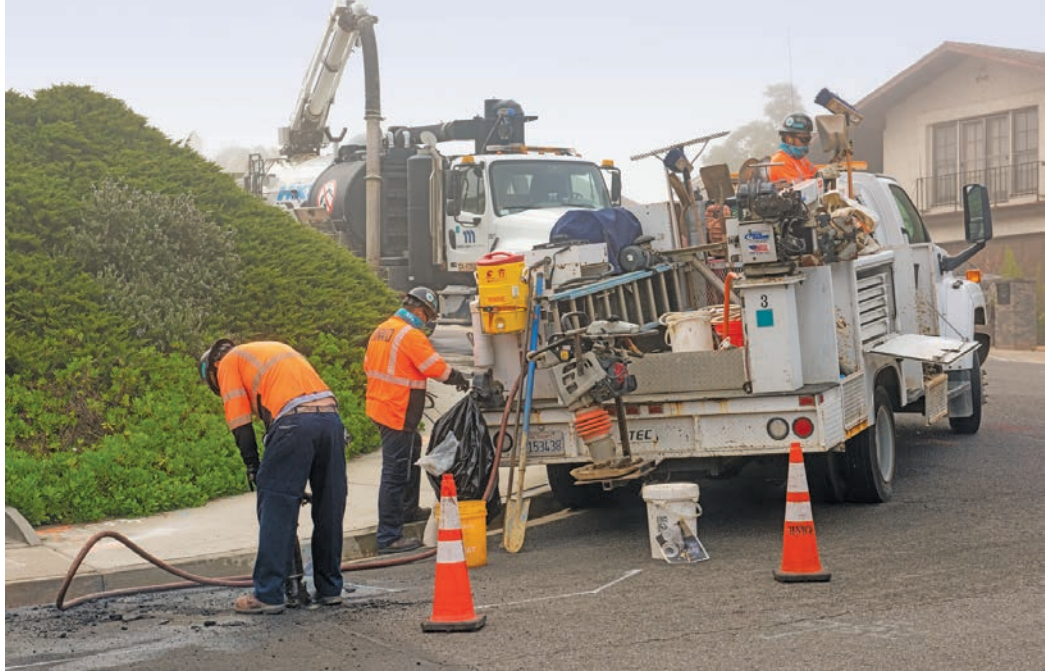
Members of the Moulton Niguel Water District blue street crew excavate a small section of pavement for a valve replacement.
