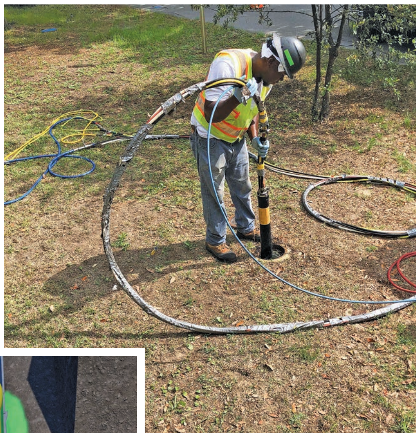
A wastewater technician launches a Logiball push-pull packer at a cleanout.
