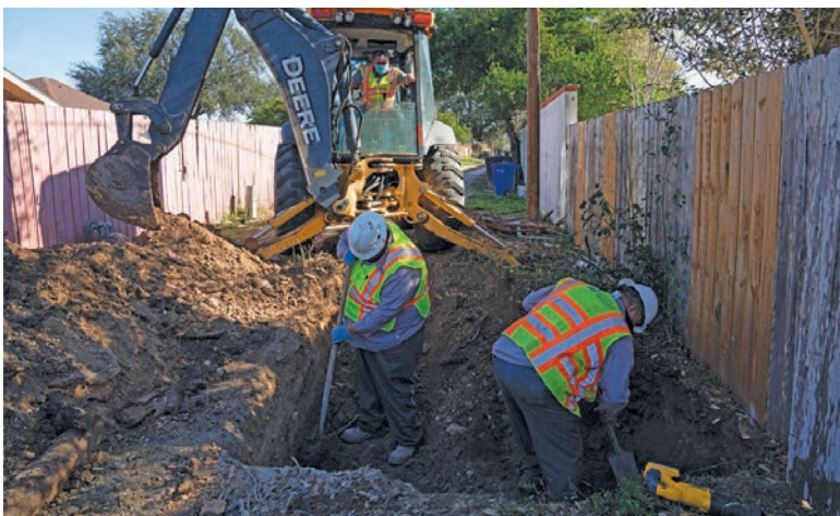
Edgar Villalpando operates a backhoe while Richard Belis (left) and Miguel Solis dig to expose a sewer lateral for repair.
