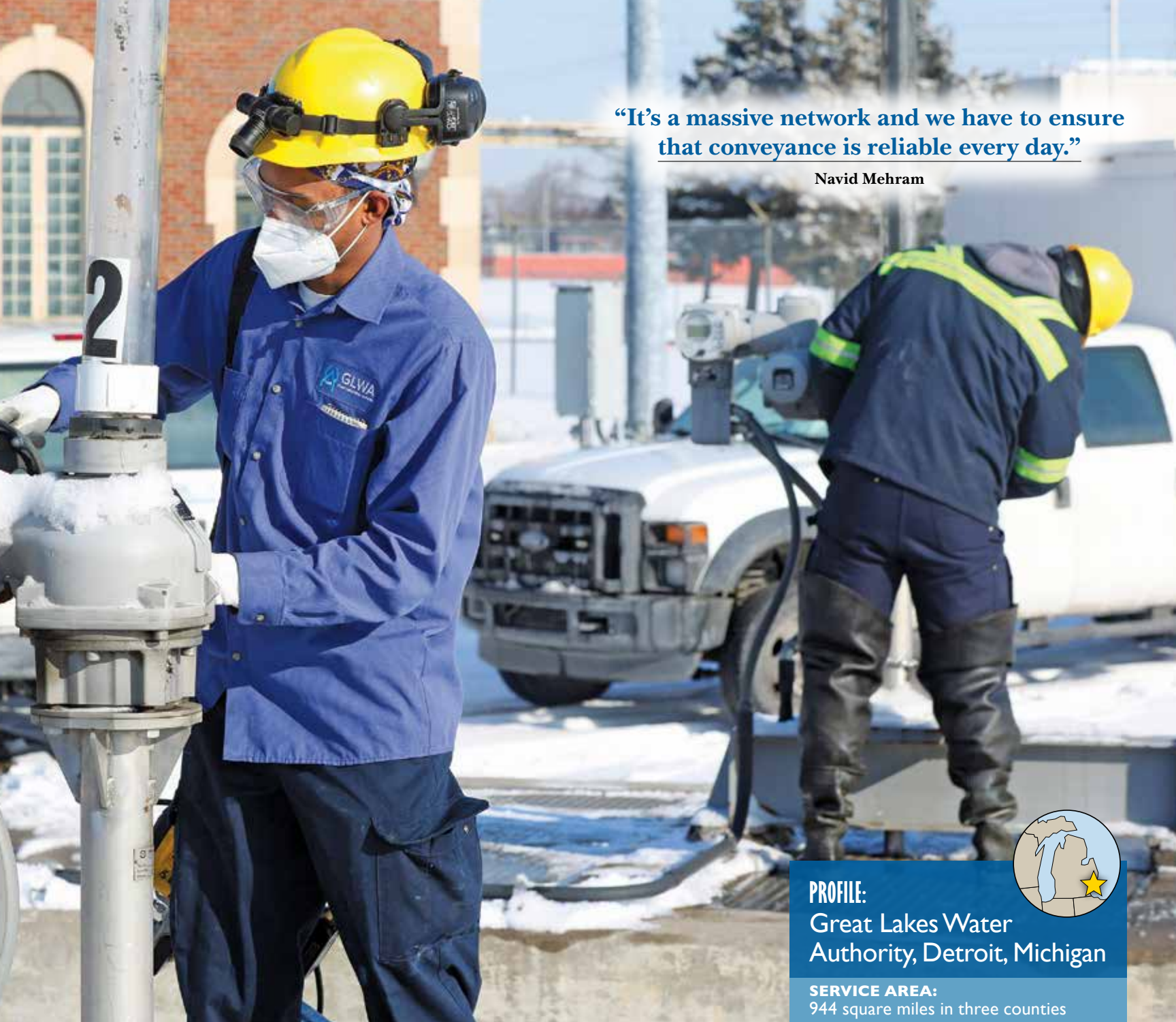
Great Lakes Water Authority maintenance technician Hawun Howard services and greases the forebay gates at the Connor Creek Pump Station in Detroit, Michigan. (Photography by Amy Voigt)
