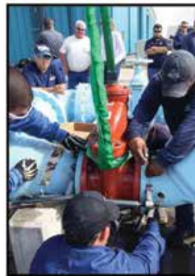
Reinstall new valve
