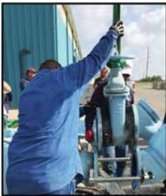
Spread outside flanges & remove old valve
