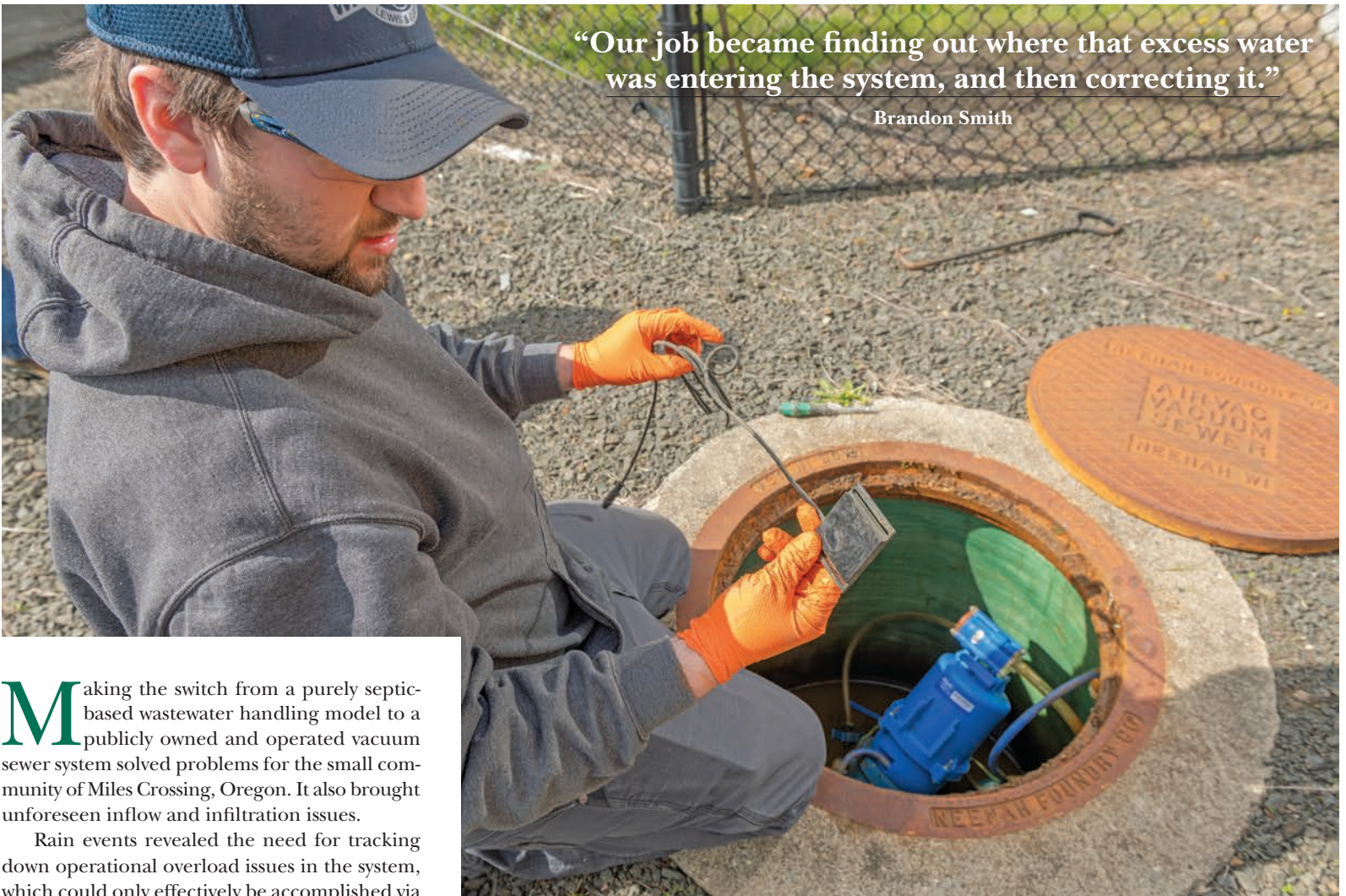
Operator Brandon Smith gets ready to install a FLOVAC valve sensor on a valve body.
