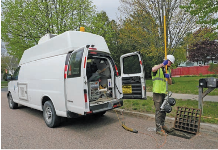
Dave Wheeler launches an Envirosight Rovver X camera into a catch basin for a storm sewer inspection.
