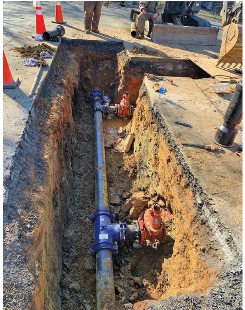
The HYMAX GRIP is a coupling restraint that can be used on several types of metal and plastic pipes. It offers continuous dynamic deflection so that the connecting pipes can flex within the coupling.
