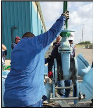
Spread outside flanges & remove old valve
