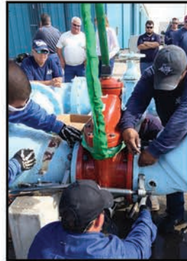
Reinstall new valve
