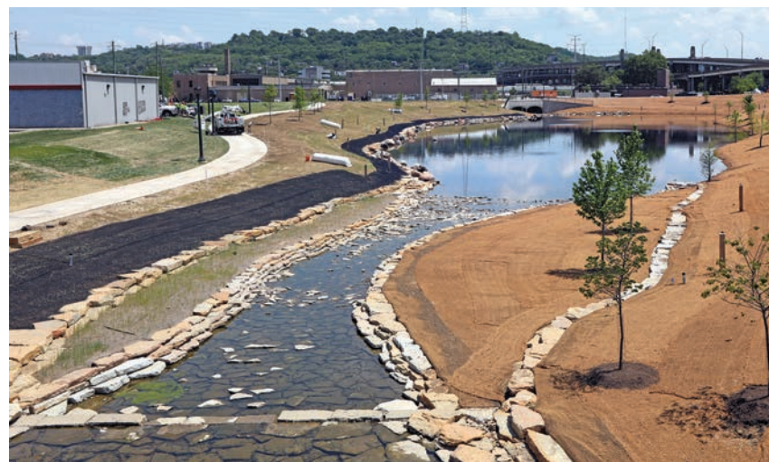
Contractors put the finishing touches on the east end of the Lick Run Greenway project, where collected stormwater flows into the pond.
