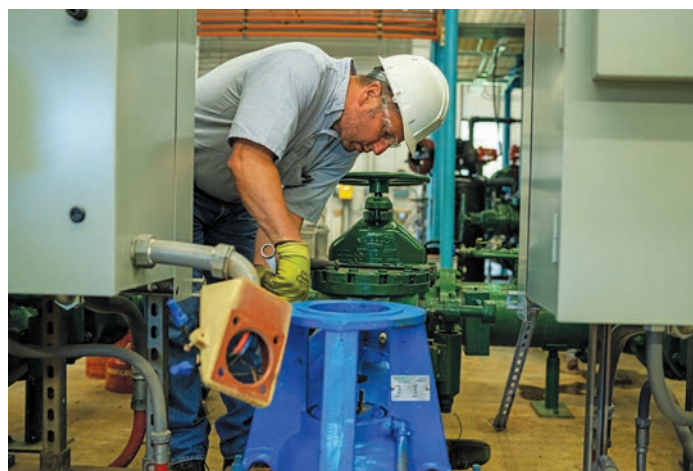
Superintendent Mike Hopf works on a raw water pump (Mueller) at the Saugerties Water Treatment Plant.
