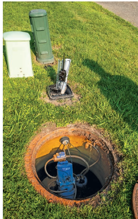
Right: A monitoring system sits outside the manhole for a residential service check valve. Each pit serves up to four homes.
