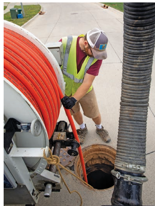
Wastewater operator Jared Keenan uses a Vactor 2100 jet/vac truck to clear a sewer line ahead of a road construction project.
