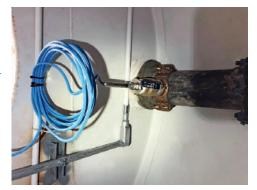
ter, can directly and accurately measure flow at the discharge side of the pump. The Mace Doppler Insert Velocity Sensor connects to the Mace Flo-Pro XCi meter and uses an I/O card to deliver flow data to the plants' SCADA systems for 24/7 monitoring and alarming. In addition, a Web-Comm card can be used for remote meter management and to transmit directly to the cloud. As many as five Doppler sensors can be monitored with a single FloPro XCi meter.
