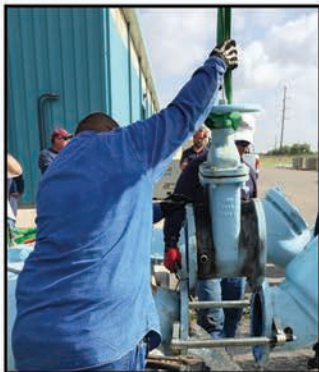
Spread outside flanges & remove old valve
