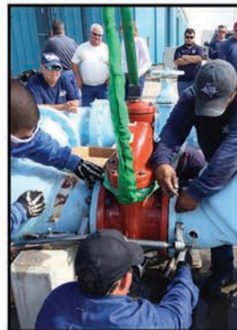
Reinstall new valve
