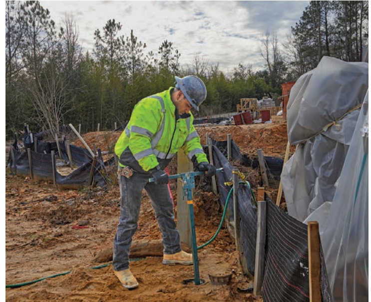
A crew member prepares a valve to relieve pressure.
