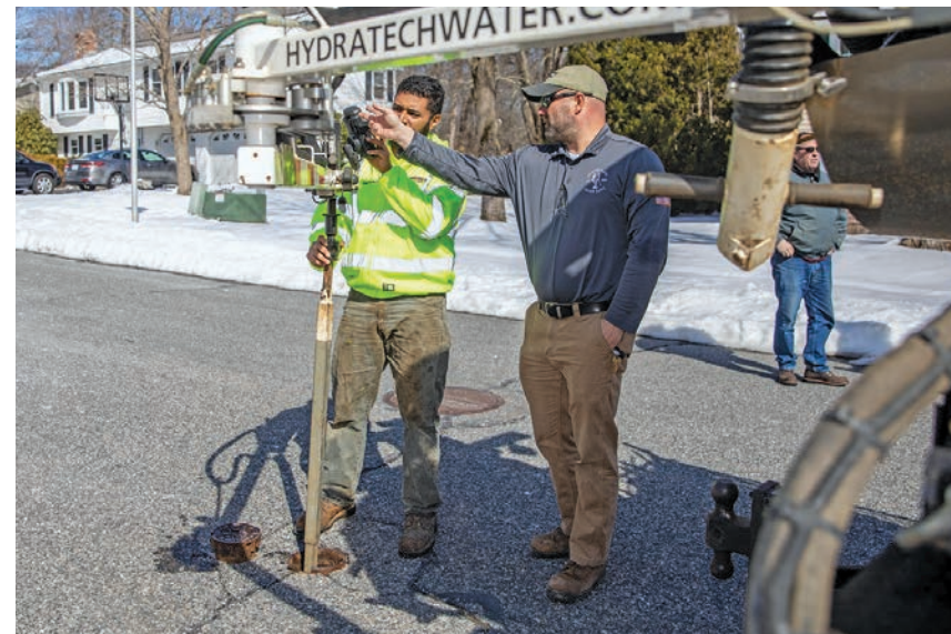
Top: Jonathan Gonzalez-Rosario exercises a water valve using a Wachs Utilty valve maintenance system in the roadway in Shrewsbury.
