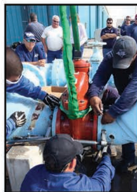
Reinstall new valve
