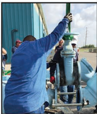
Spread outside flanges & remove old valve
