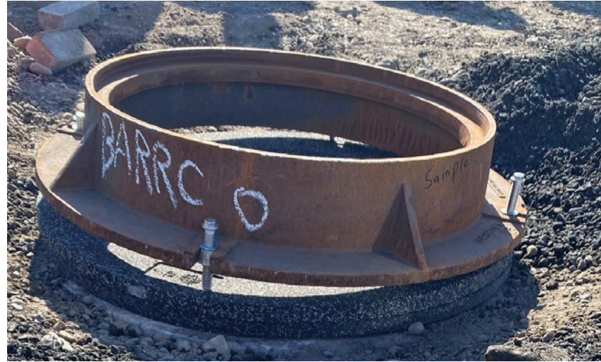
Screw-adjusted systems like RimRiser ensure manholes and catch basins are set correctly.
