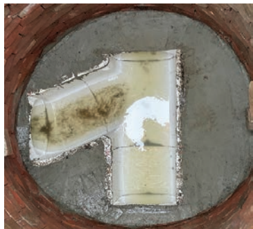
RELINER/Duran Manhole Invert Channel
