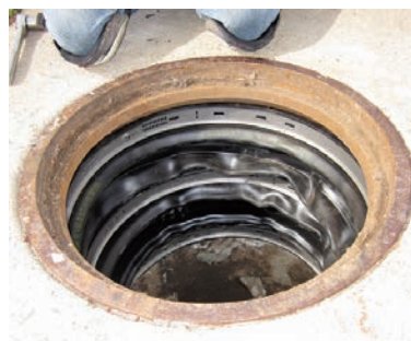
Cretex Specialty Products Internal Chimney Seal
