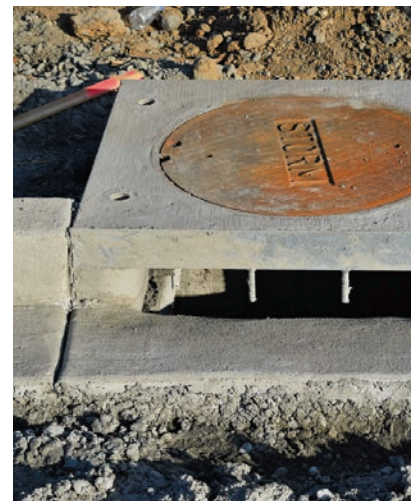
Screw-adjusted systems like RimRiser ensure manholes and catch basins are set correctly.
