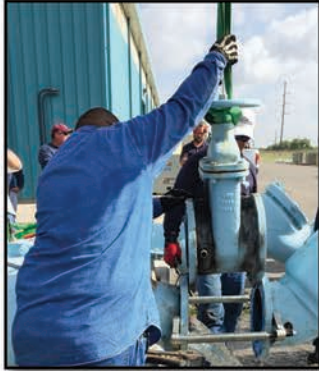
Spread outside flanges & remove old valve
