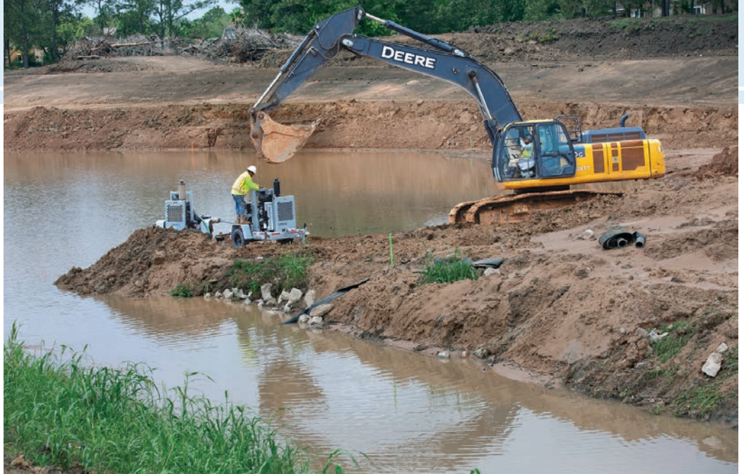
Above: Jose Banderas and Elder Arana from Serco Construction Group move a 3-inch water pump from Lance Rentals to remove stormwater from a Clear Lake City Water Authority construction site.
