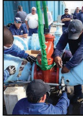
Reinstall new valve
