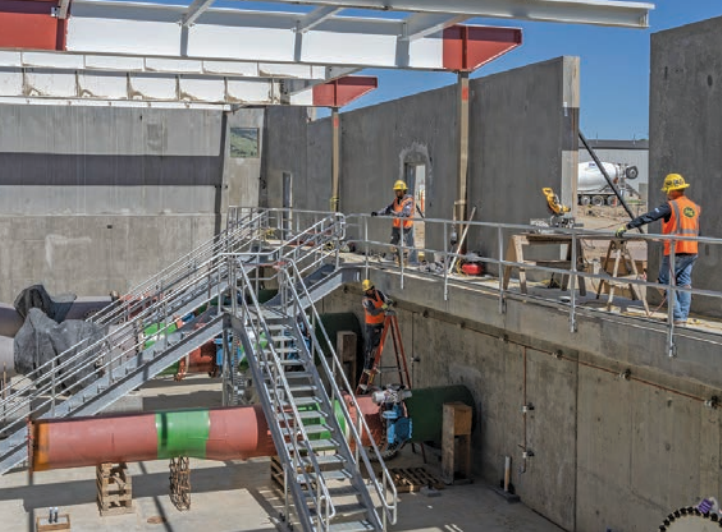
A construction crew works at the water intake and hydro-electric generator room in the filters building.
